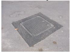
North Somerset CC has five antiskid inspection covers to be trialed on North Somerset's roads, the first of which has now been installed in Nailsea on a sharp bend.
