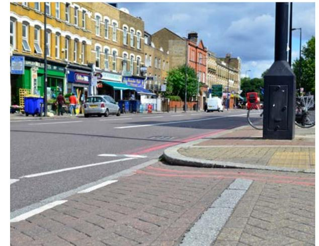
*The up ramp starts directly at the border with the main carriageway at the point where the motorcyclist will start the turning manoeuvre. There is also a change in road surface at this location.*
