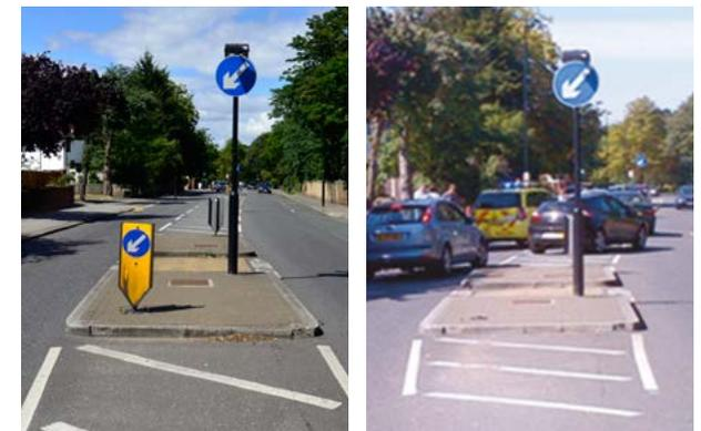
*These two pictures show the same refuge, one with a low-level keep left bollard and the other where the bollard is missing. The missing bollard increases the risk of a vehicle striking the refuge, particularly at night or in bad weather.*
