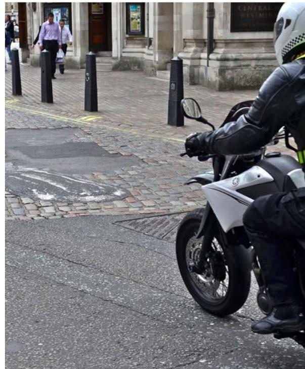
*Here there are four different road surfaces within close proximity. Tarmac, inspection covers, worn thermoplastic on a raised oval of tarmac (with no warning) and cobbles. In an area with a high pedestrian flow and busy traffic lanes, this will cause stability problems for motorcyclists.*
