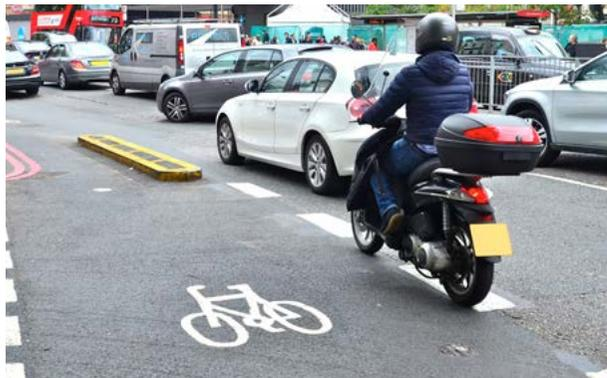
*The kerbed island is not easy to identify (no bollards or other features) and forms a collision hazard for motorcyclists.*
