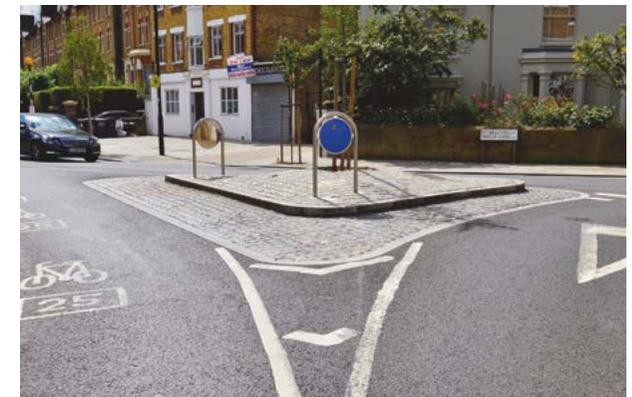
*The cobbled overrun area in this picture is in an area where motorcycles may be leant over, and could be slippery when wet. Also the white lines may guide motorcycles into the cobbled area at night, rather than around it.*
