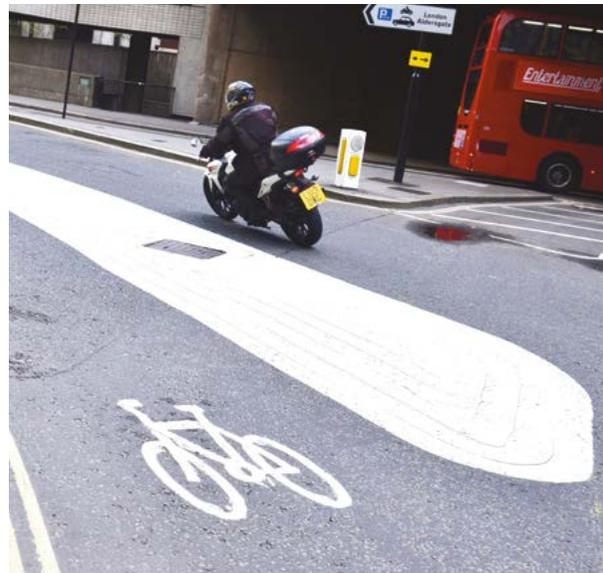
*The photograph shows a sharp bend with a large area of thermoplastic segregating the cycle lane from the traffic lane. This could present a loss of control hazard for motorcyclists, particularly when the road surface is wet.*
