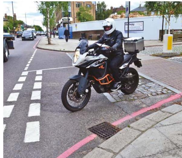
*The braking area on the approach to the junction has a granite sett down ramp, which is poorly maintained and has substandard reinstatement where it has been repaired.*
